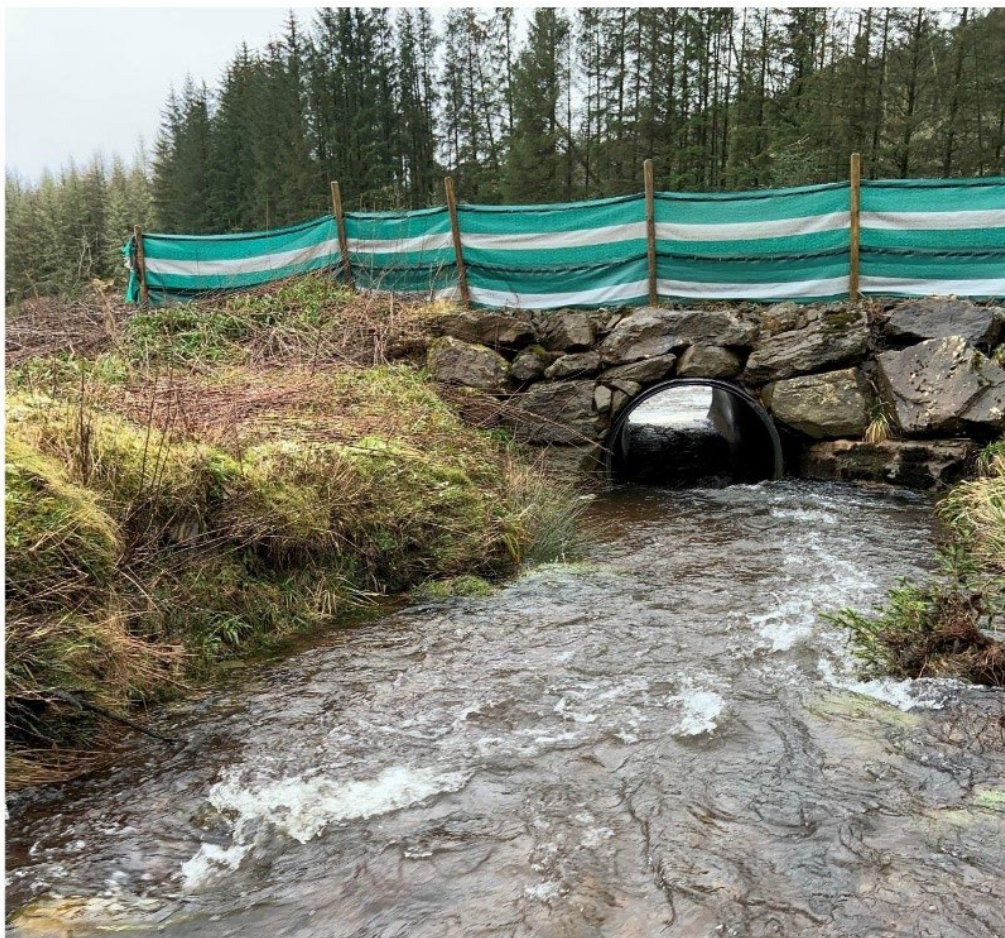
Plate 3.5: Silt Fencing at Watercourse Crossing
