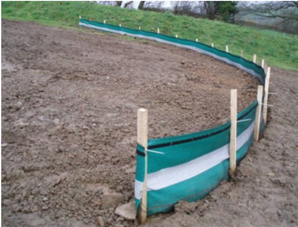
Plate 3.5: Silt Fencing at Watercourse Crossing
