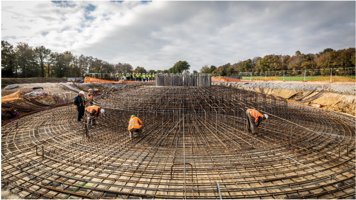
Figur 18. Gravitationsfundament.
