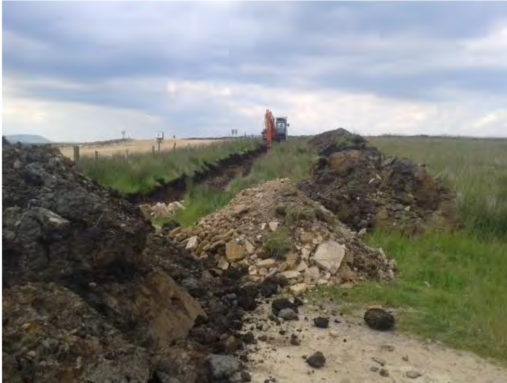
Plate 3.2: Stockpile and drainage ditch (under construction)
