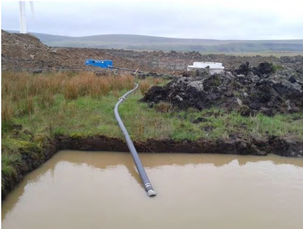
Plate 3.8: Settlement lagoon and Siltbuster pumping out water for treatment
