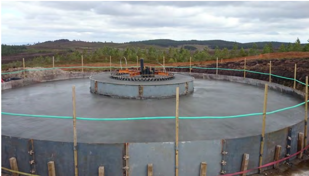
Plate 3.12: Shuttering for concrete foundation (wind turbine base)
