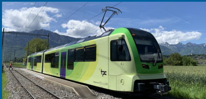
Chablais: modernisation with electronic interlockings for TPC
