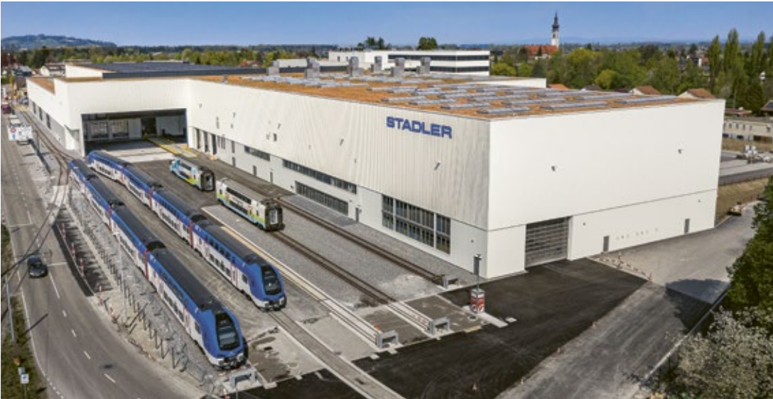
After a construction period of two years, Stadler moved into the new production plant in St. Margrethen
