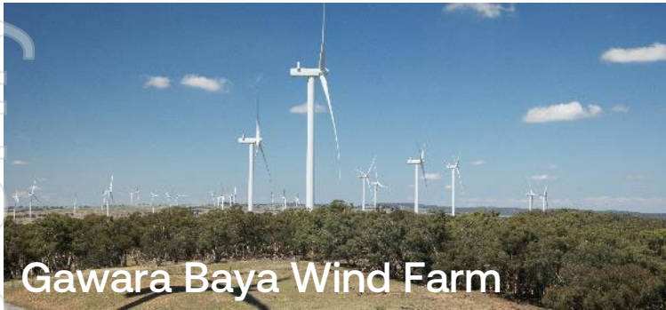
Gawara Baya Wind Farm ECI complete, main project awarded to Symal (1)
