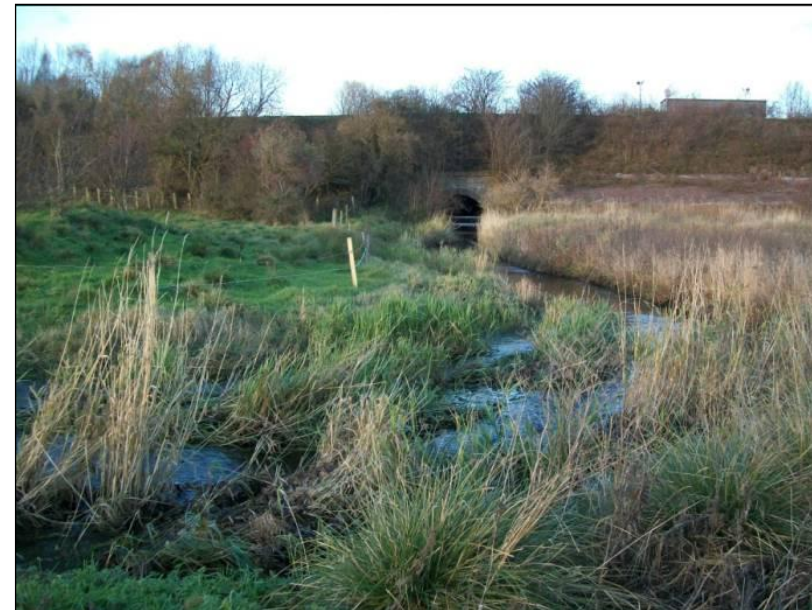
Bothlin Burn flowing into railway culvert
