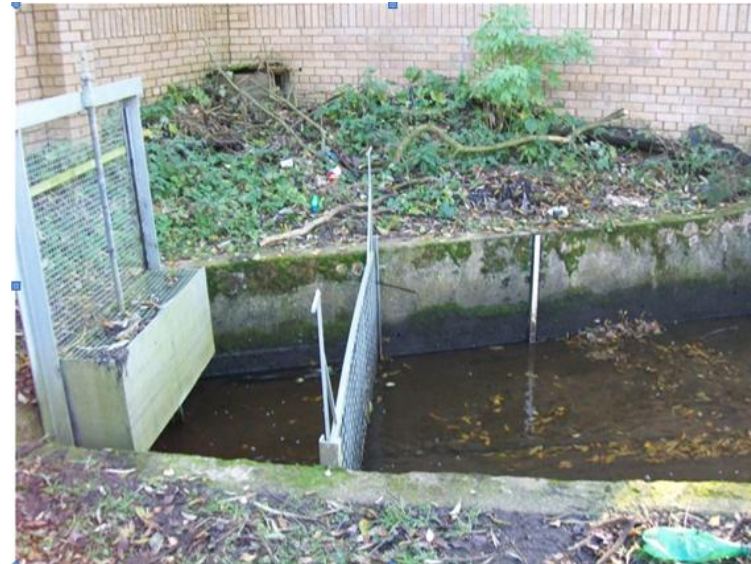
Figure 17: Sluice Gate at Lochend Loch
