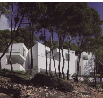
Hillside dwellings, Alvaro Siza, Portugal
