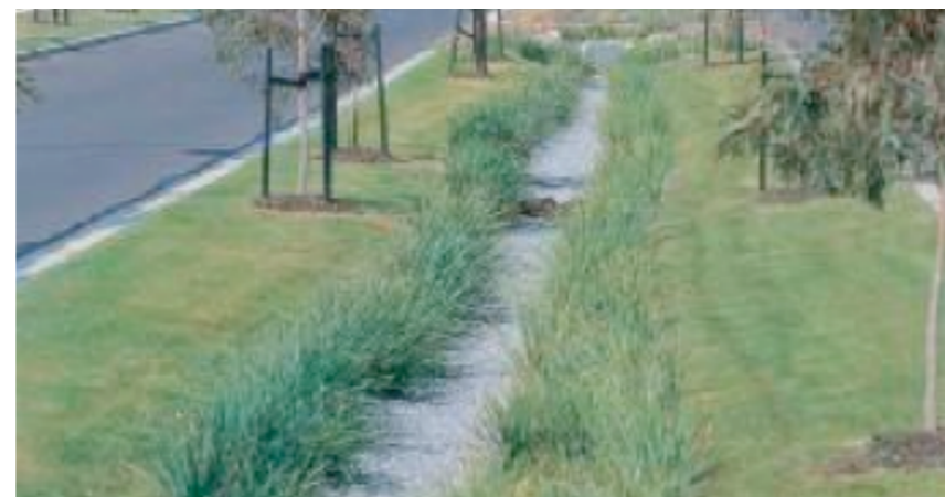
example of linear wetland within a central reservation
