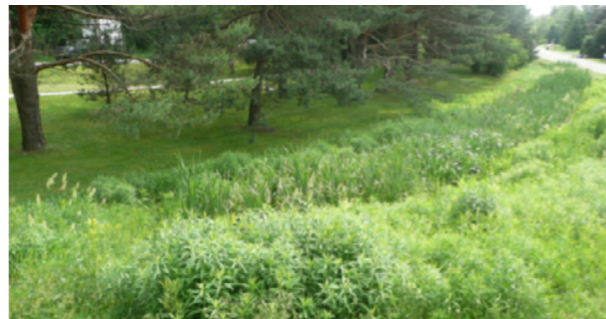
example of a drainage swale
