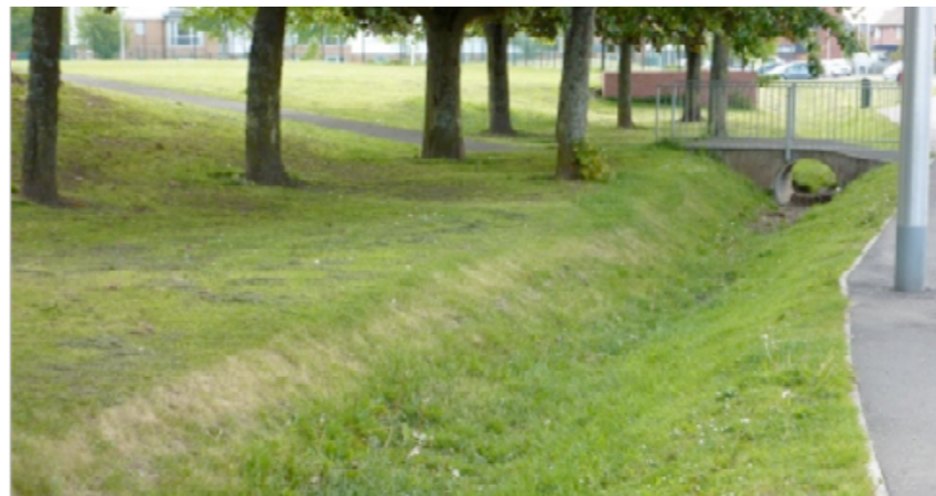
example of a swale
