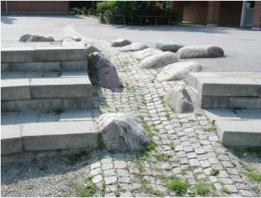
Water conveyance, Malmö, Sweden
