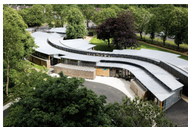
Hazelwood School, Glasgow, UK
