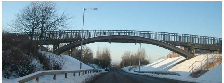
Existing Greenhills Road
