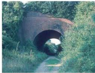
Path reinstatement under bridge
