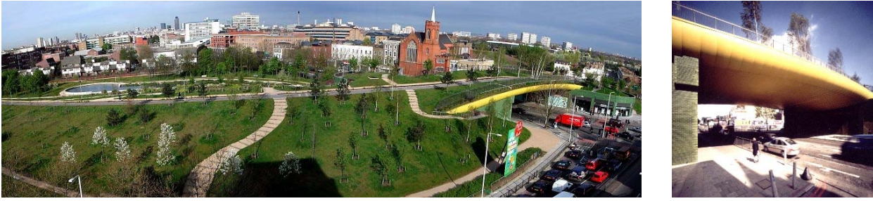
Figure 5.4: 'Green' Bridge (Grassed) at Mile End Park, London, Joining Sections of the Park Over Busy Road
