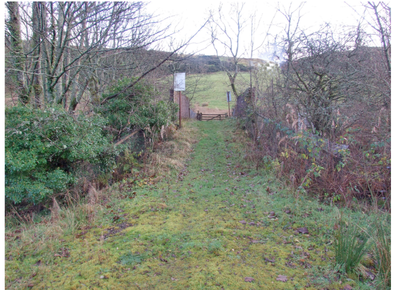
access over rail line
