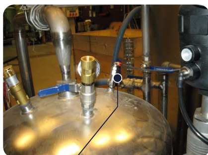
Picture 1. Non-return valve ¼" (no. 137) Article no. 16101
