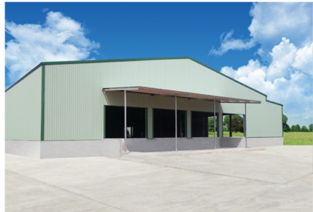
Mangoteen Warehouse - Chantaburi
