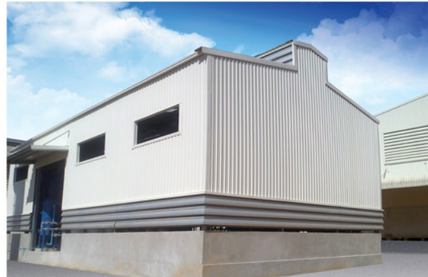
Ligman Warehouse - Chachoengsao
