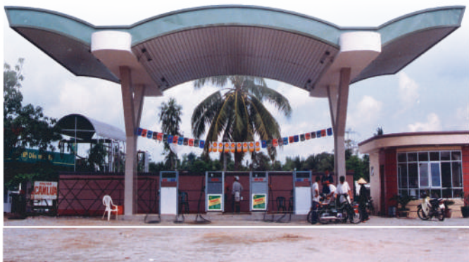
Trạm xăng – Petrol Station
