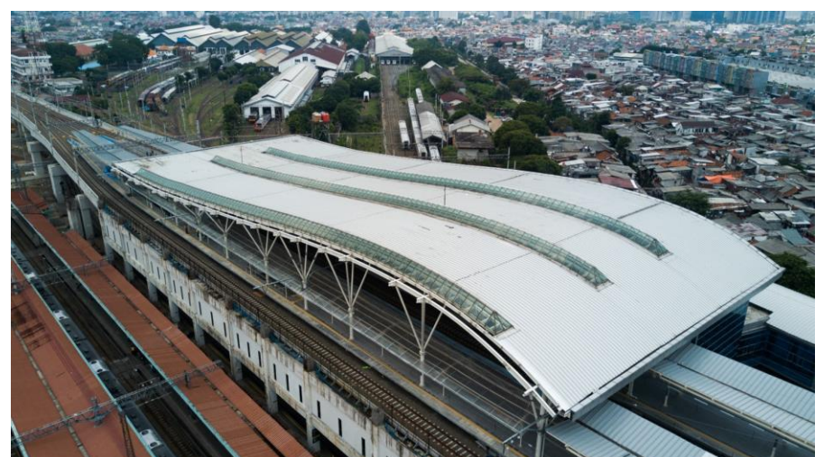
Manggarai Station is using LYSAGHT® FLEXLOK® COLORBOND® Gull Grey produced using Mobile Rollforming and On-Site Curving method.
