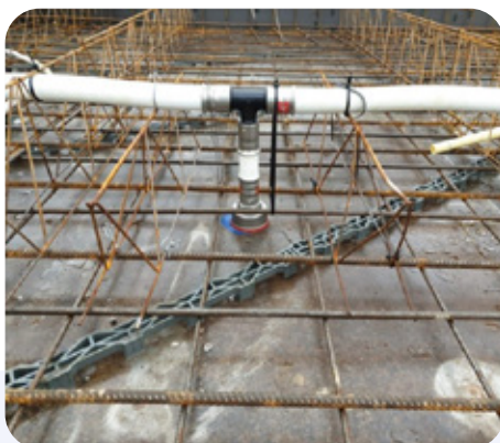
50P sprinkler holder glued to metal formwork
