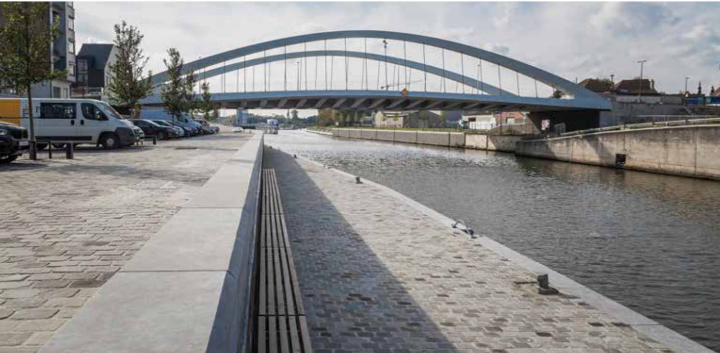
Oriental Basalt, Kandla Grey - cleft - Lys River Copings, Harelbeke (BE) kerbstones: Belgian Blue Limestone - sanded
