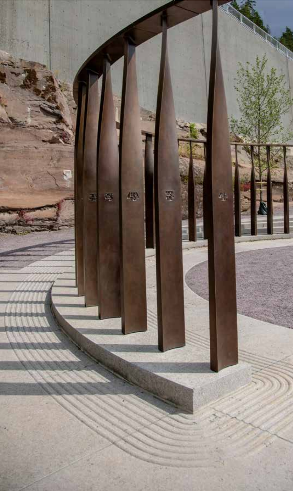
Blue Antique - bush hammered and sandblasted - The National Memorial in Utøya (NO)
