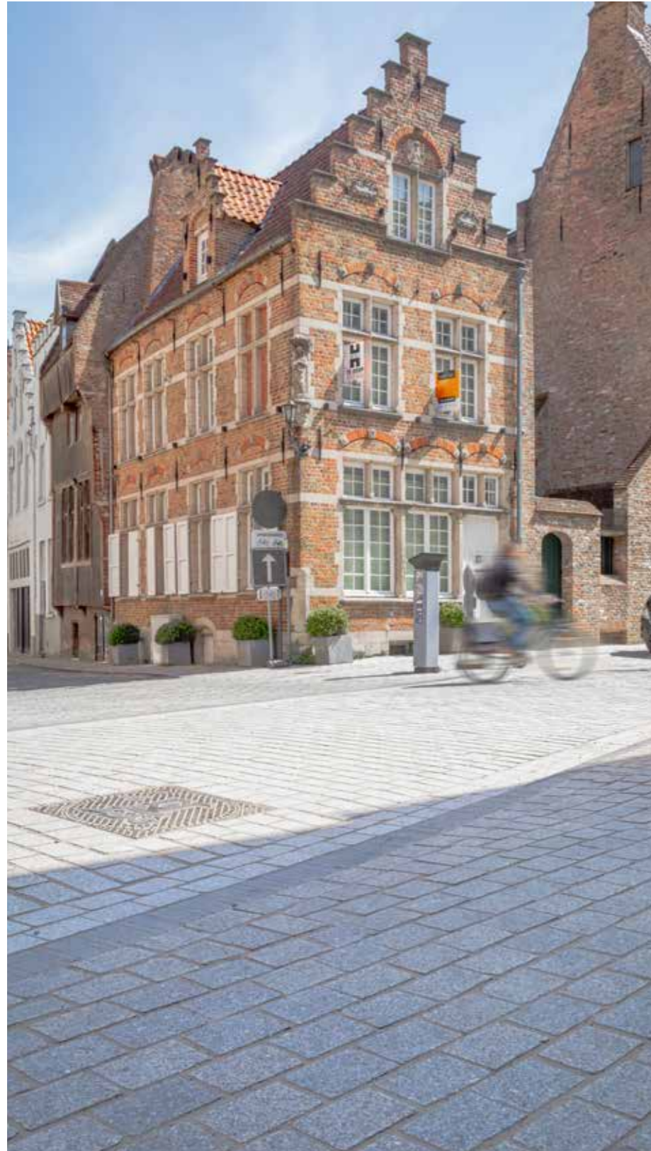
Azul Platino - flamed - Vlamingstraat, Bruges (BE) kerbstones: Kilkenny Limestone - line chiseled street: Tarn - flamed surface and cleft edges
