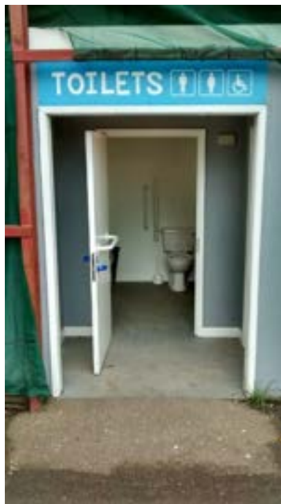
Accessible toilet. Other toilets to the left and right.
