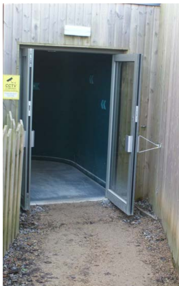
Entrance to Time Chamber and Bear Wood
