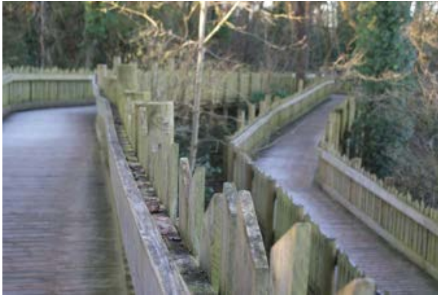
Wooden walkways through Bear Wood
