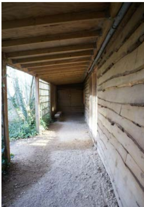
Ringtail Lemur viewing area with seating.
