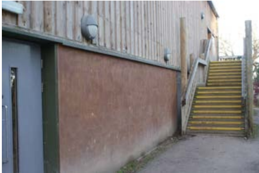
Door to downstairs viewing on left and steps up to the higher viewing area
