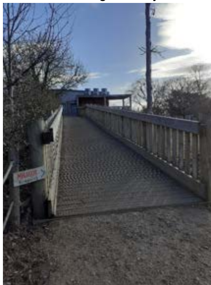
Ramp up to the higher viewing area of Giraffe House
