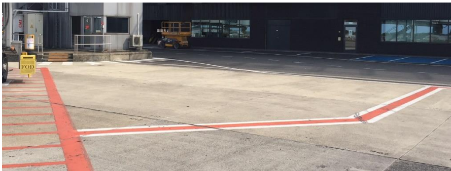
Fig. 14. Equipment staging area
