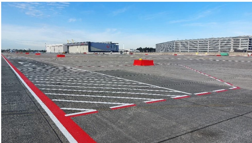
Fig. 15. Staging area op de power-in power-out stands
