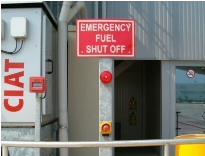
Fig. 58. Noodstop brandstofhydrant
