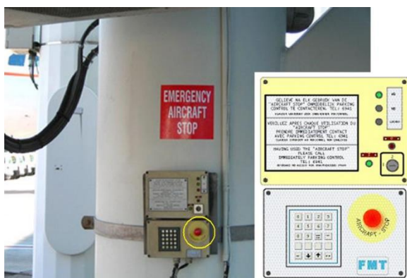
Figure 54: DGS Emergency stop Pier B, level tarmac
