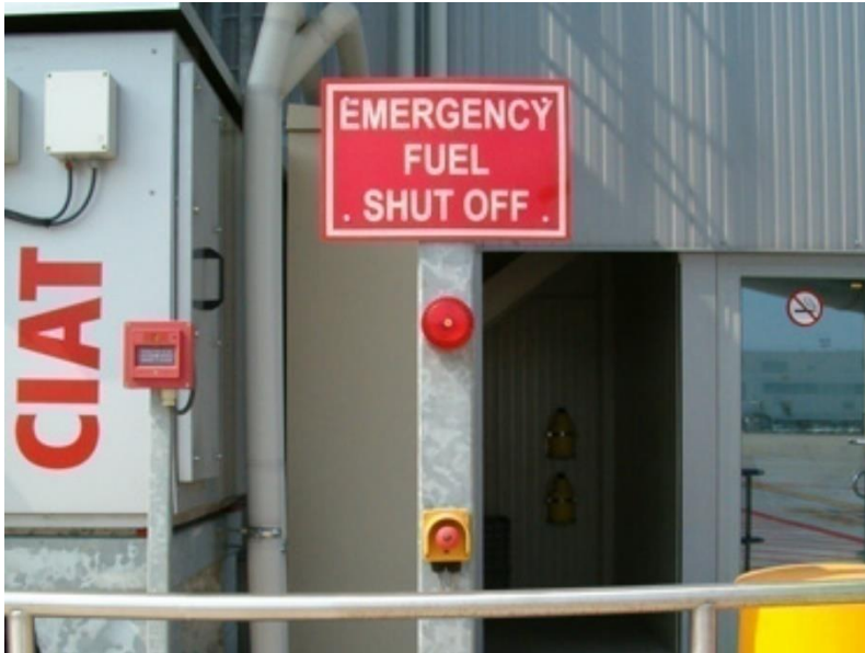
Figure 58: Emergency stop fuel hydrant
