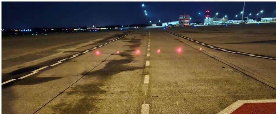
Fig. 9. Service drive stop bar
