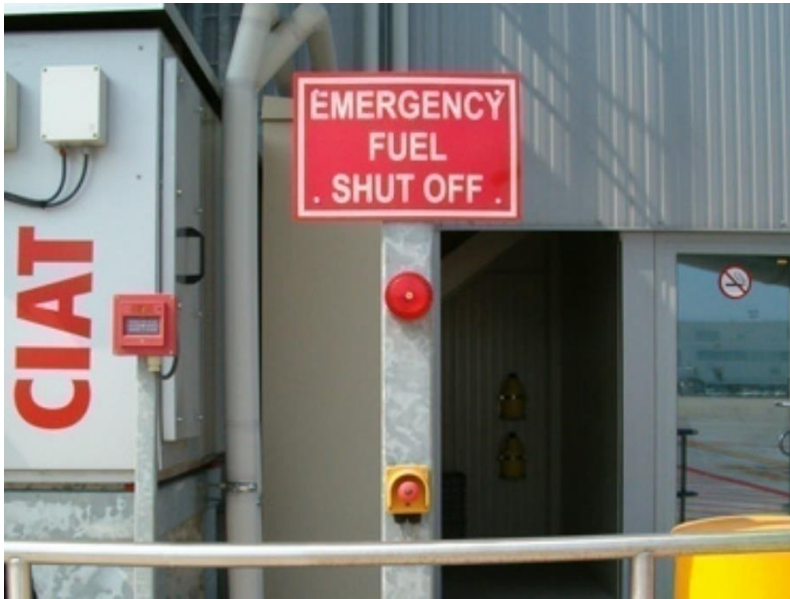
Fig. 57. Noodstop brandstofhydrant
