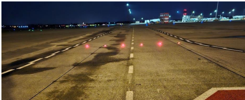
Fig. 10. Service drive stop bar
