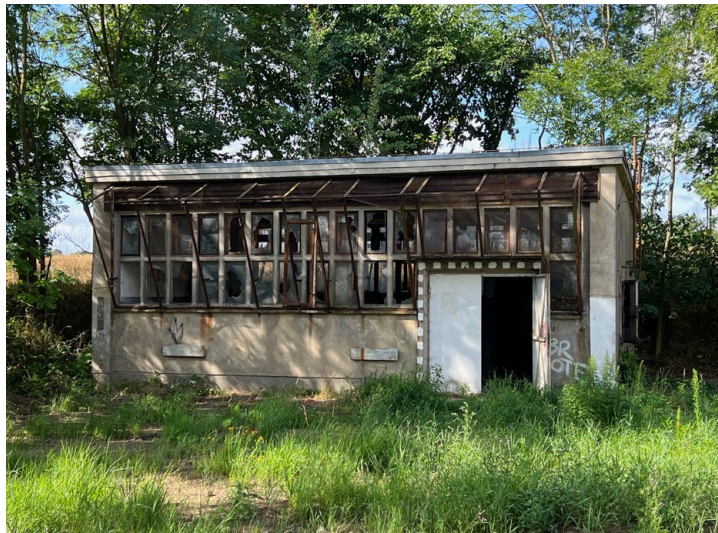
Former gas regulator station
