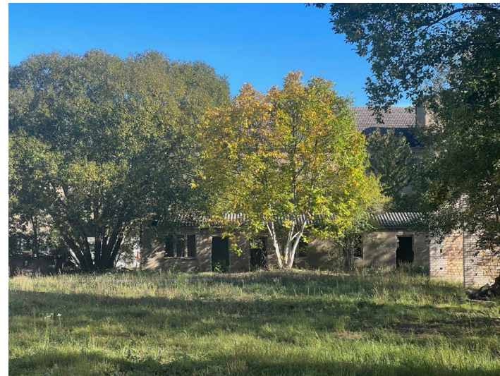
Former office spaces
