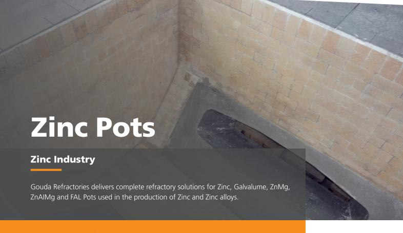
For many years, Gouda Refractories has successfully designed and supplied refractory materials for pots for different types of Zinc alloys. Due to the close relation with our customers, Gouda Refractories is strongly involved in the development of suitable refractory lining for new alloys.
