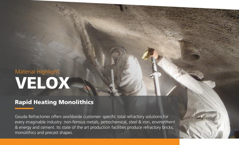
Special range of Velox monolithics for repair and maintenance purpose. Velox monolithics don't require a long curing and dry-out curve and are therefore excellent materials for short shut-downs were the dry-out cannot be performed within a standard heating time frame.
