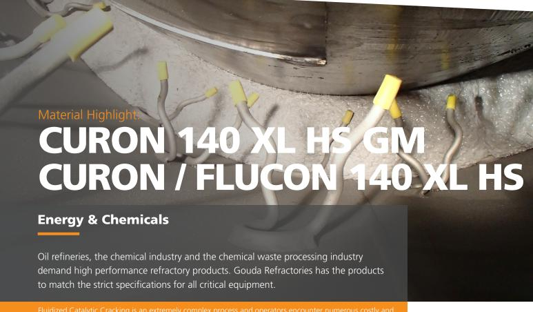
Fluidized Catalytic Cracking is an extremely complex process and operators encounter numerous costly and difficult problems. For Flue gas / Transfer lines and ducts, the challenge is to develop an insulating castable with abrasion resistant capabilities. Gouda Refractories can now add to its FCC material series a new castable with maximum density of 100 lbs/ft³ (1.600 kg/m³) and a maximum Erosion Loss (EL) of 20 CC according to ASTM C704/C704M.
