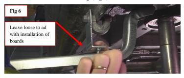
**Step 7:** Next install the Middle Front (Tallest & Longest). Obtain one of the bolt plates and insert it into the hole as shown.
