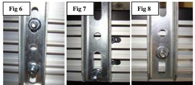
There are several configurations to mount the boards to the brackets. We have provided some suggestions in the figures above. These changes allow you to adjust the board in or out according to your step preference. All are correct.
