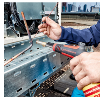
Brazing in refrigeration / air-conditioning technology
