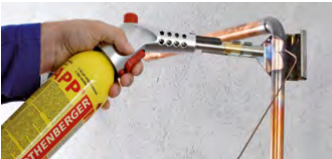
Brazing in gas installation
