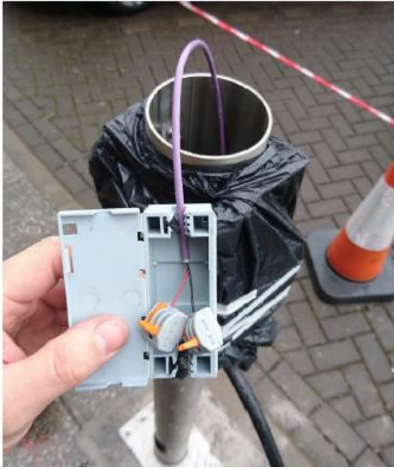
Figure 3 - Wago or Lever style connectors
