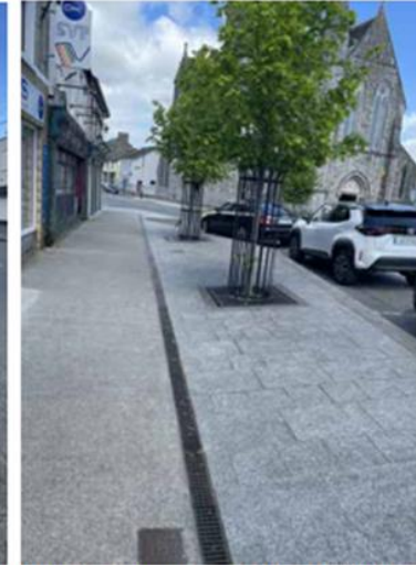
Street Drainage - Attenuation and retention features can be added to roadside drainage systems for greater sustainability in streetscapes.
