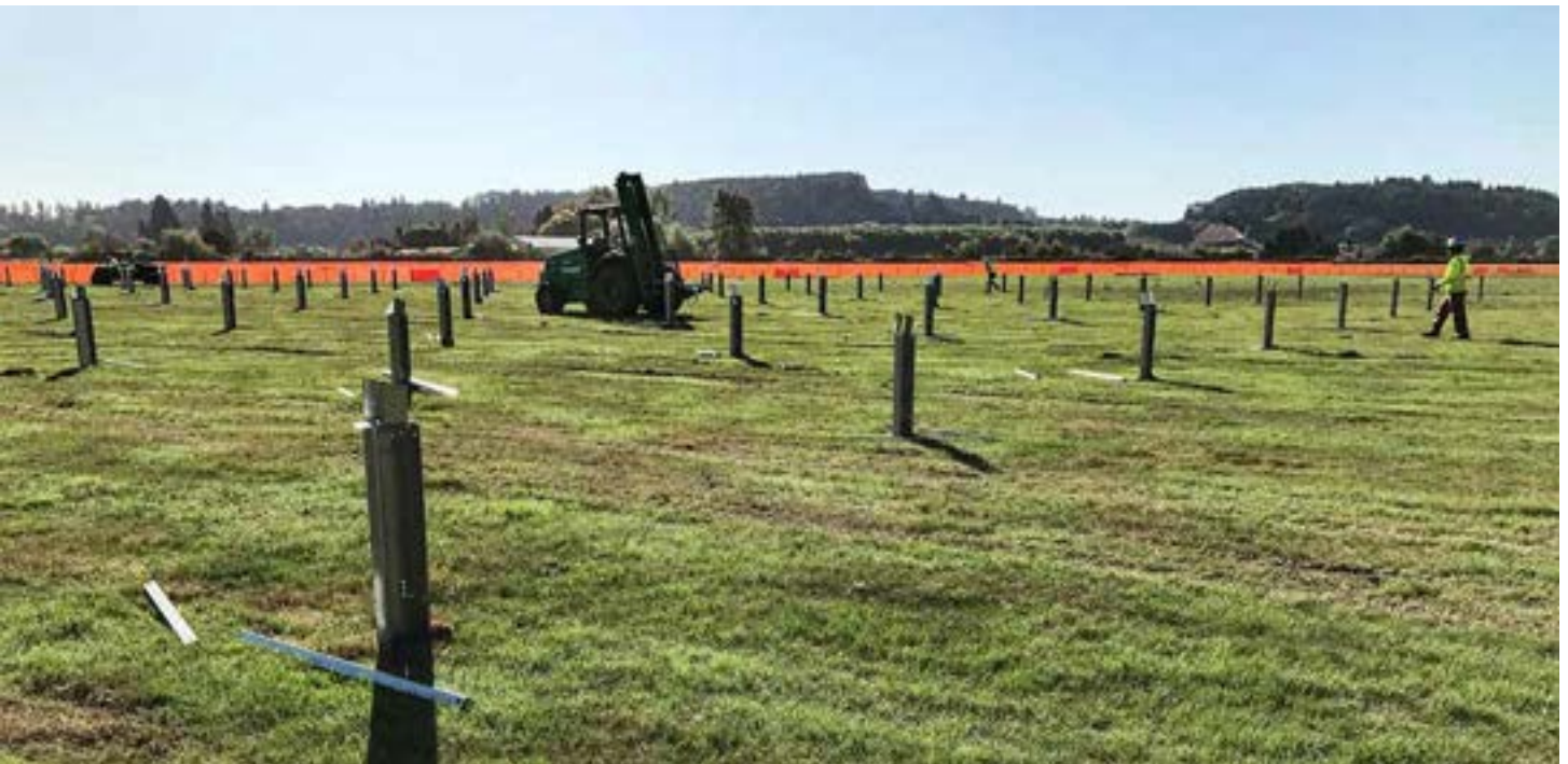
Solar site preparation and construction developed around existing vegetation, Photo by Jordan Macknick, InSPIRE project principal
