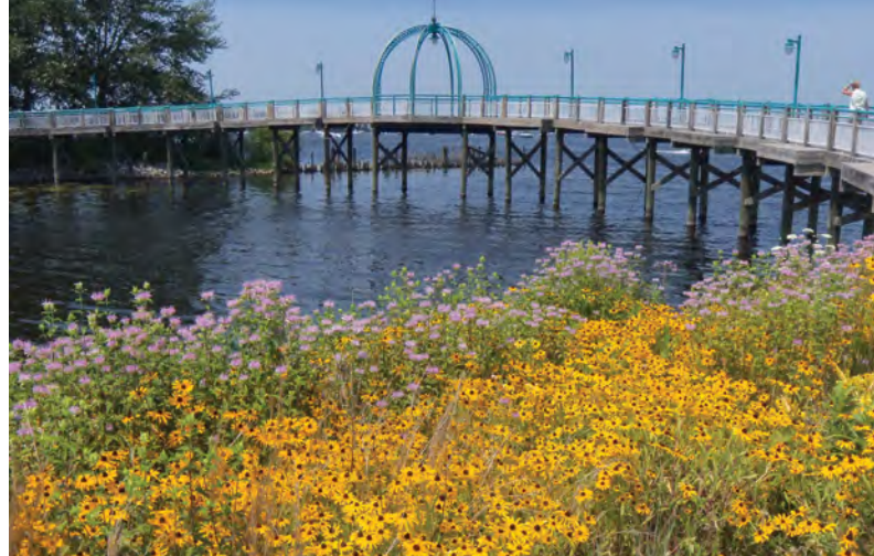
Lake Muskegon shoreline. Photo: GEI Consultants
