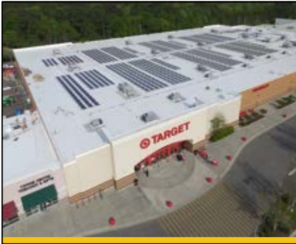
Hannah Solar North Charleston Site.
