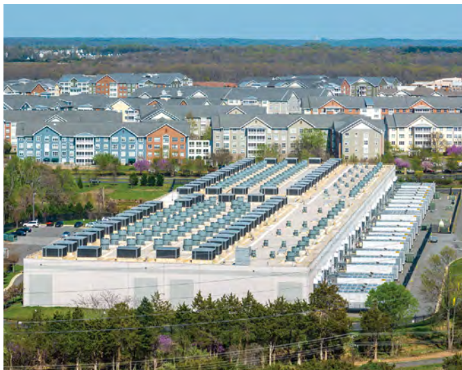
↑ A data center close to homes in Loudoun County, Virginia.
