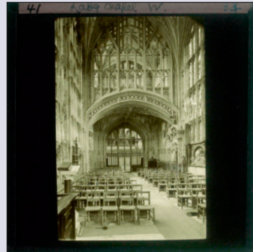
Lantern slide showing the Lady Chapel with Gurney stove to provide heating, c.1900
