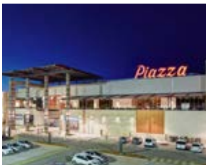
Sanliurfa Piazza shopping mall Sanliurfa, Turkey - 1 Water source heat pumps SYSHRW
