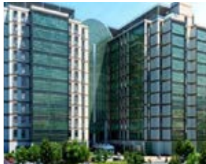
Vizyonpark shopping mall Istanbul, Turkey - 3 Water source heat pumps SYSHRW
