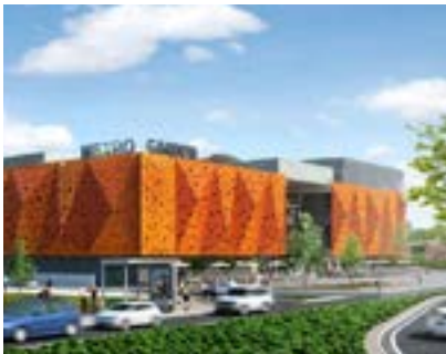
Metro Garden shopping mall Istanbul, Turkey - 2 Water source heat pumps SYSHRW
