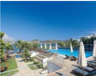
Milpoint Hotel Muğla, Turkey - Hotel - Air cooled chiller SyScroll 280 Air EVO - Total capacity 280kW
