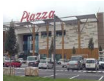
Mara Piazza shopping mall Kahramanmaraş, Turkey - 2 Water source heat pumps SYSHRW
