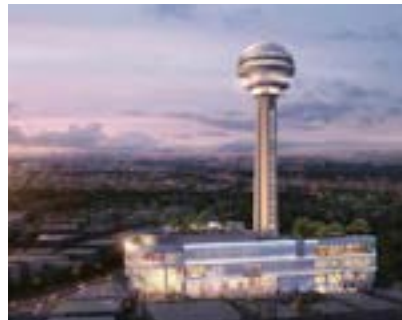
Atakule tower Ankara, Turkey - 209 Water source heat pumps SYSHRW
