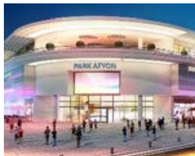
Park Afyon shopping mall Afyonkarahisar, Turkey - 3 Water source heat pumps SYSHRW
