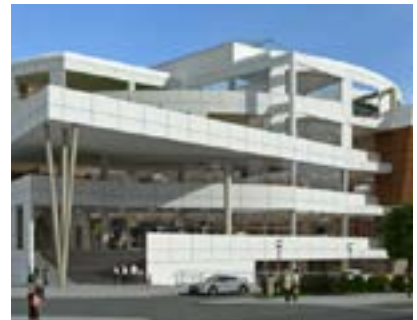
Corlu Trend Arena shopping mall Tekirdag, Turkey - 19 Water source heat pumps SYSHRW
