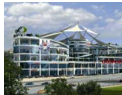
Otoport shopping mall Istanbul, Turkey - 1 Water source heat pumps SYSHRW
