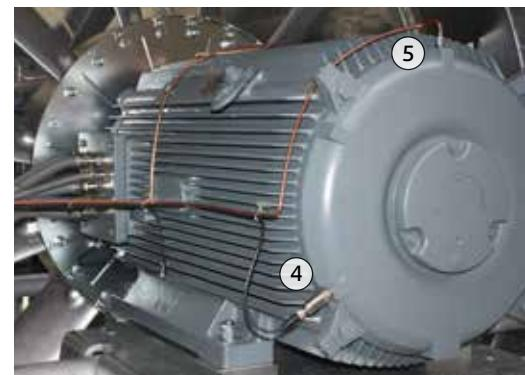
Vibration sensor (4), regreasing pipework (5) to DE + NDE bearings.
