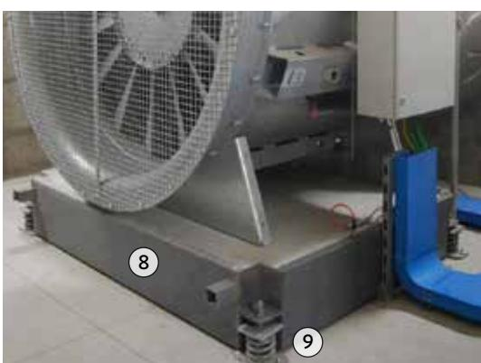
Base frame (8), spring vibration isolators (9)
