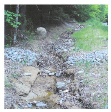
The proposed project addresses an area of the road between Deer Run and Hazard Cove Road. The work will improve culvert and ditch conditions that are currently causing soil erosion. In addition to the work outlined on the grant application, the Penobscot County Soil & Water Conservation District made additional recommendations for work that should be included in the project to more fully address and correct the issue.
